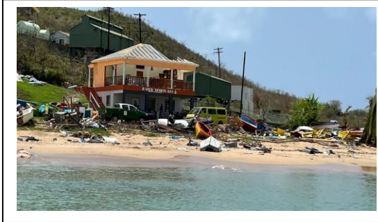
Picture 6: Visual of damages in Mayreau, coastal
