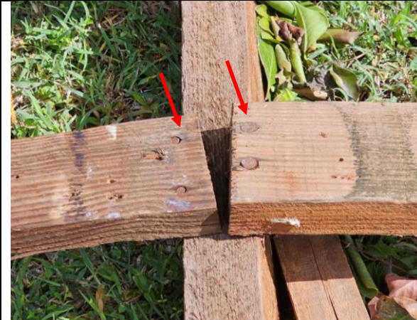
Inadequate end distance (nail to end of timber). It should be minimum 7 times the nail diameter.
