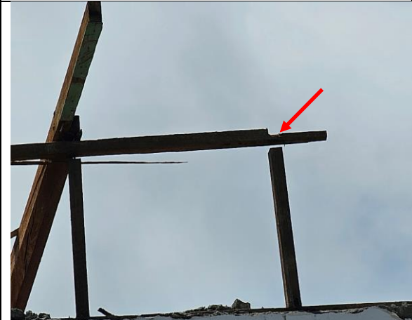
Inadequate end distance (nail to end of timber). It should be minimum 7 times the nail diameter.
