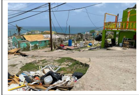
Picture 7: Visual of damages in Mayreau, interior
