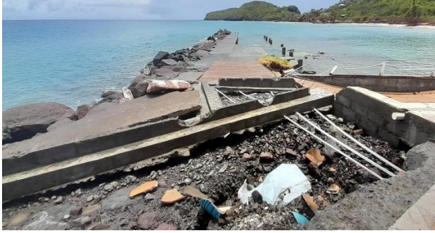
Top: Damaged deck and pier at The Liming Bottom: Part of Damaged Roof at The French House
