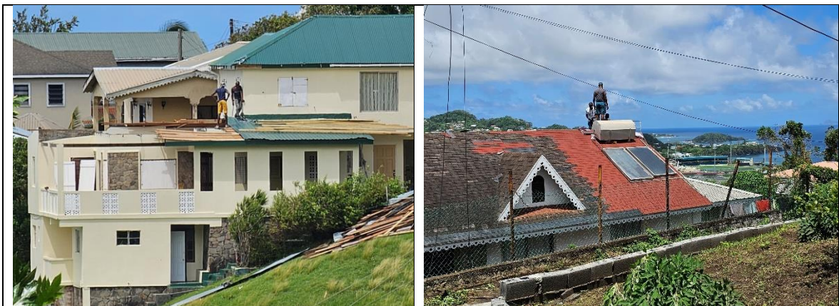
Figure 12 - Rebuilding started (4 July 2024).
