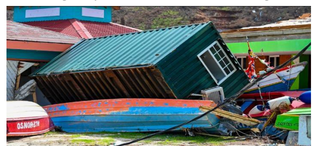
Damaged Water Taxis
