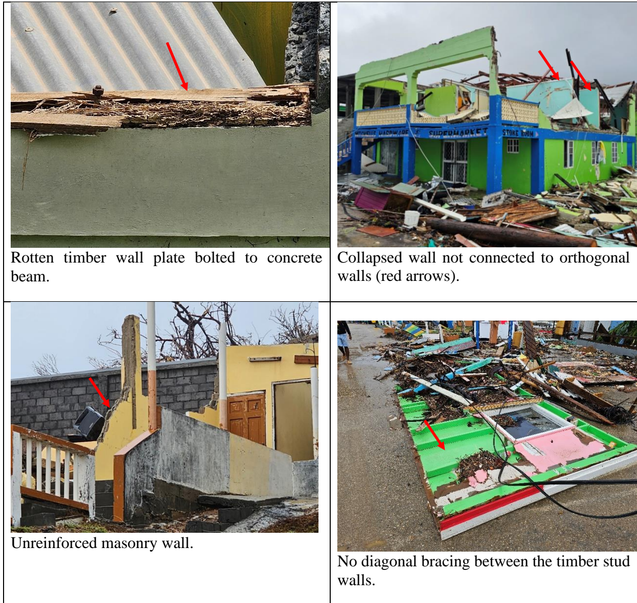
Figure 9 – Roof frame failure modes.
