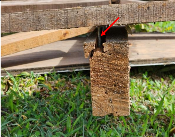
Inadequate edge distance (nail to edge of timber). It should be minimum 4 times the nail diameter.
