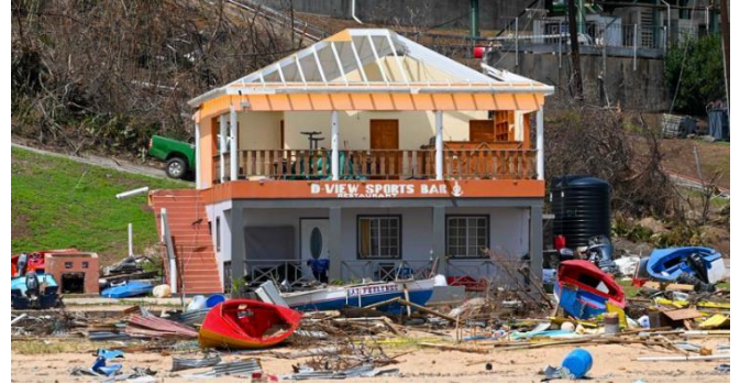
Saline Bay – Damaged Boats, Bars and Restaurants
