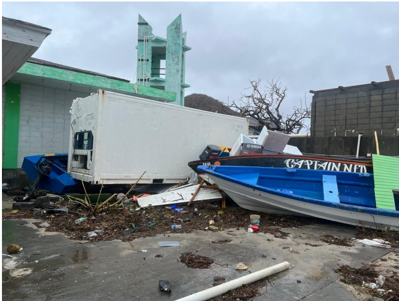
Union Island. Cold storage and fishing boats dislodged and damaged.
