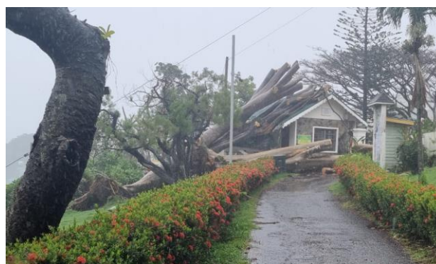
Fallen Tree on Visitor Centre at Botanic Gardens
