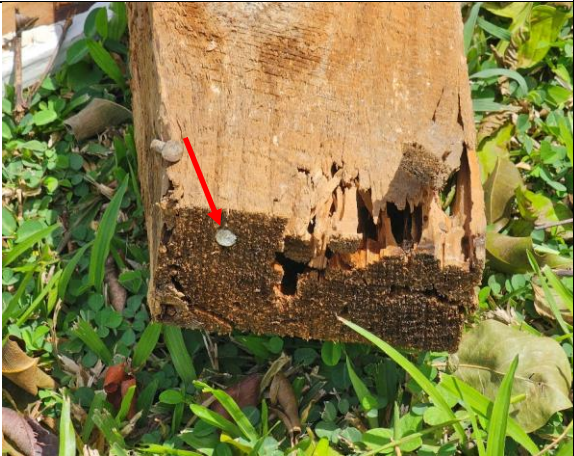
Inadequate edge distance (nail to edge of timber). It should be minimum 4 times the nail diameter.
