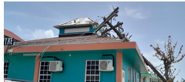
Tobago Cays Marine Park Office Building
